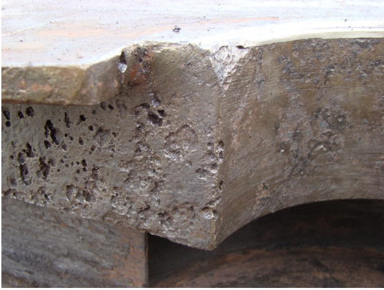
Corrosion detail
